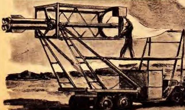
The rocket frame (on a truck) awaits inflation of the plastic balloon.
